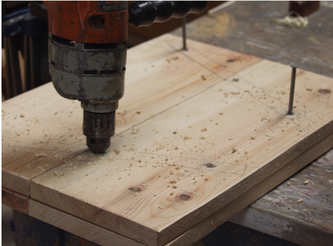
Nails dropped into screw holes maintain positioning while drilling clearance and bolt holes.
